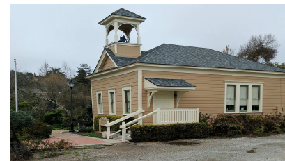
SANTA MANUELA SCHOOLHOUSE
